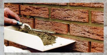
The gaps between the clinker tiles are grouted, allowing you to give the surface the appearance of perfect brickwork, as well as keep the heat inside the house. Insulated Brick Façade Panels suggest the possibility of mounting on various surfaces and all types of walls, regardless of the season.
