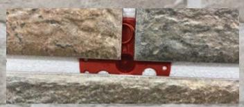
After completing the installation of the first row, proceed to the mounting of the second row, also starting from the corner of the building. The joint between the panels of the first and second row must be sealed with the PU foam as well.
