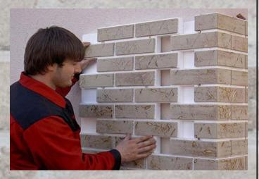
All joints between the panels are recommended to be fixed with polyurethane foam. After completing the installation of the first row, proceed to the mounting of the second row, also starting from the corner of the building. The joint between the panels of the first and second row must be sealed with the PU foam as well.
