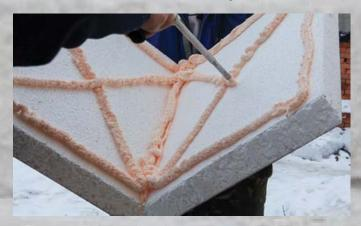
Then continue to install the wall panels. All joints between the panels are recommended to be fixed with polyurethane foam.
