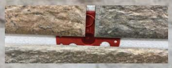
After completing the installation of the first row, proceed to the mounting of the second row, also starting from the corner of the building. The joint between the panels of the first and second row must be sealed with the PU foam as well.
