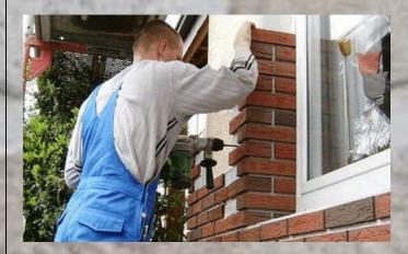
The Panels are fixed with screws in the manufacture installed pins.
